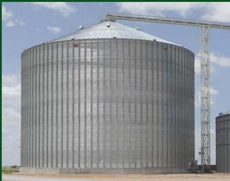
We'd only need two! Recently erected in Kansas it's the world's largest grain silo and at 37m high it holds 30,000t which can be unloaded at 270t per hour – nice.
